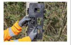
Place each enclosure support on the support plate, observing the mounting direction. Secure them by inserting the fixing pins.
