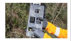
Insert the third enclosure support. Secure it with 4 fixing pins.
