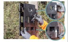
**3a MMEB 2**: Secure the two enclosure brackets with the fixing pins.
