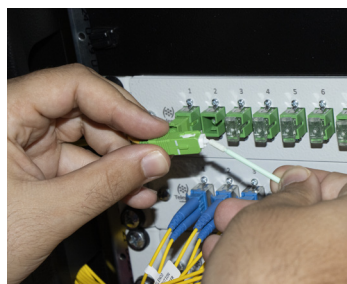
Cleaning a 2.5mm SC/ST/FC ferrule
